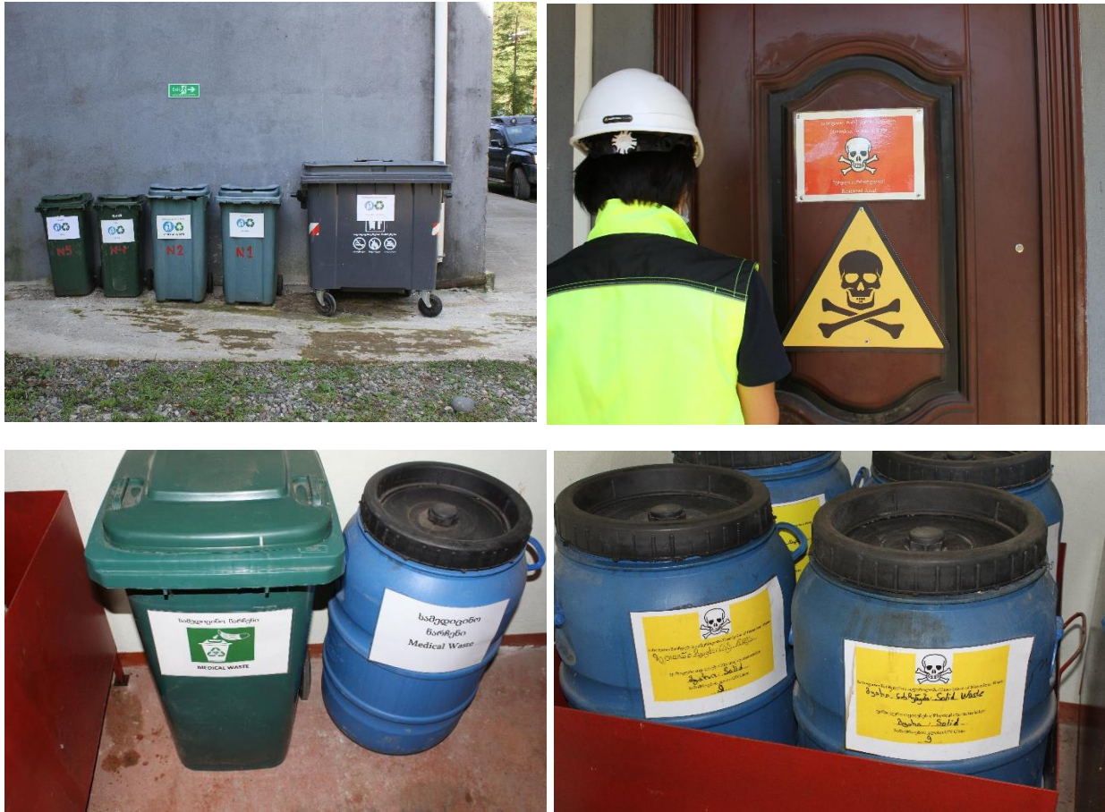
Figure 3.2: Waste segregation and hazardous materials and waste store with secondary containment at the Bakhvi 3 project during the site visit.
