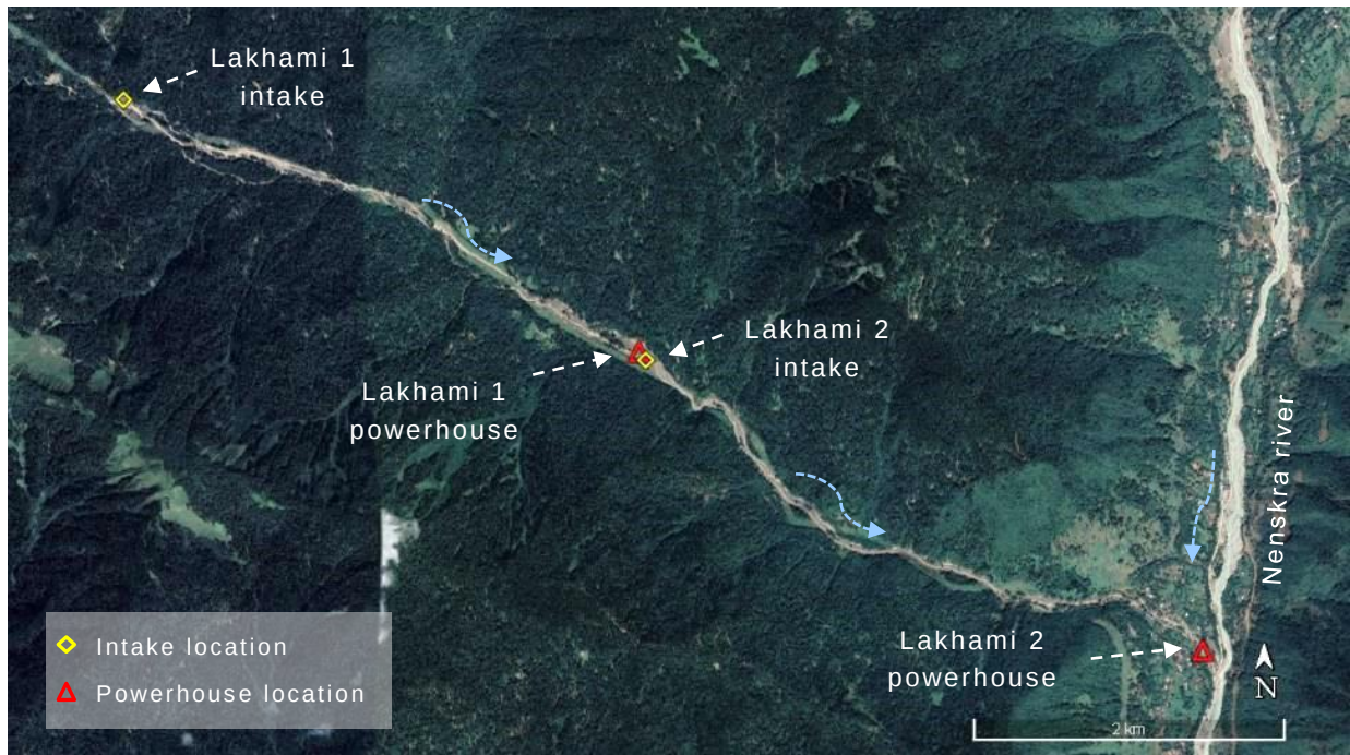
Figure 2.3: Lakhami 1 and 2 project locations (operational) on Lakhami river shortly upstream of the confluence with the Nenskra river.
