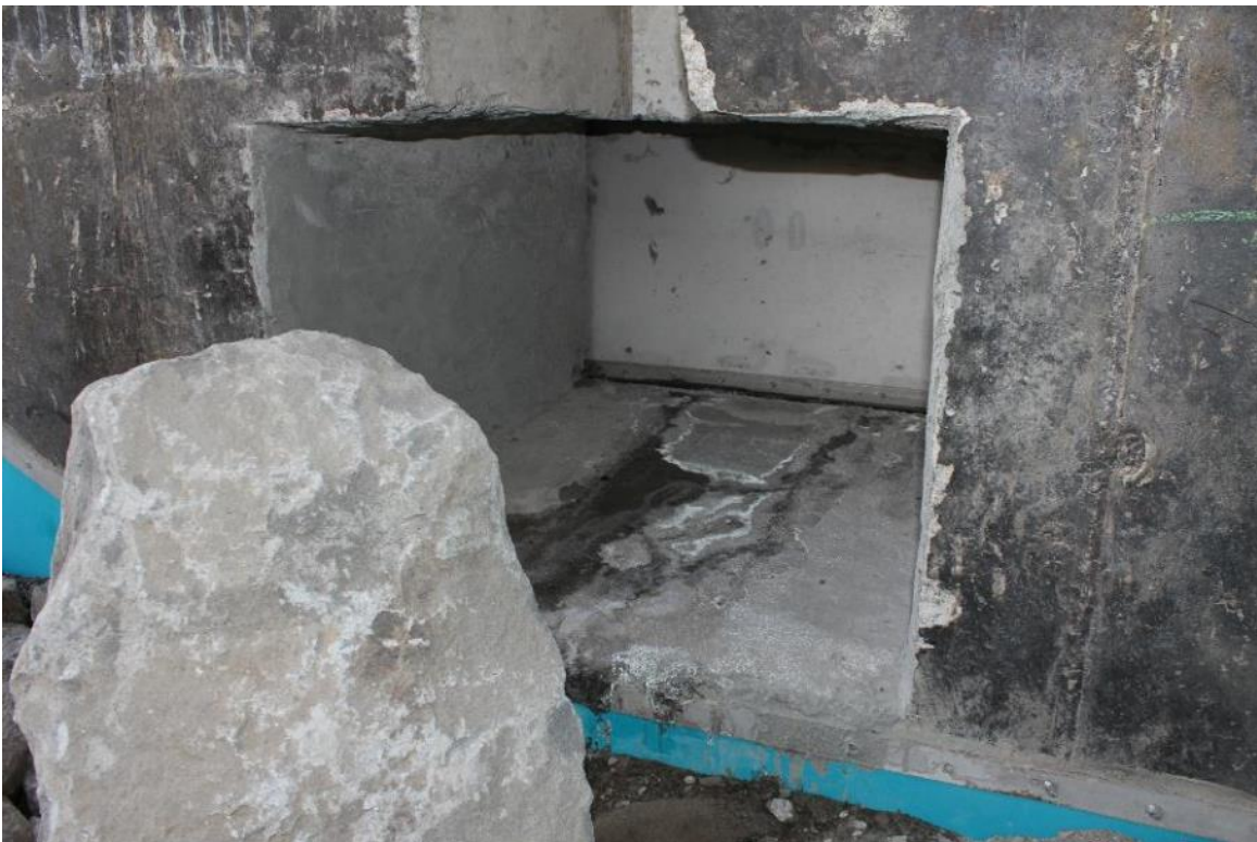
Figure 3.11: The exit at the upstream fish passage at Akhalkalaki 1, which require checks to ensure this is passable by fish due to pressurised flow (ref. also Figure 3.7 above).
