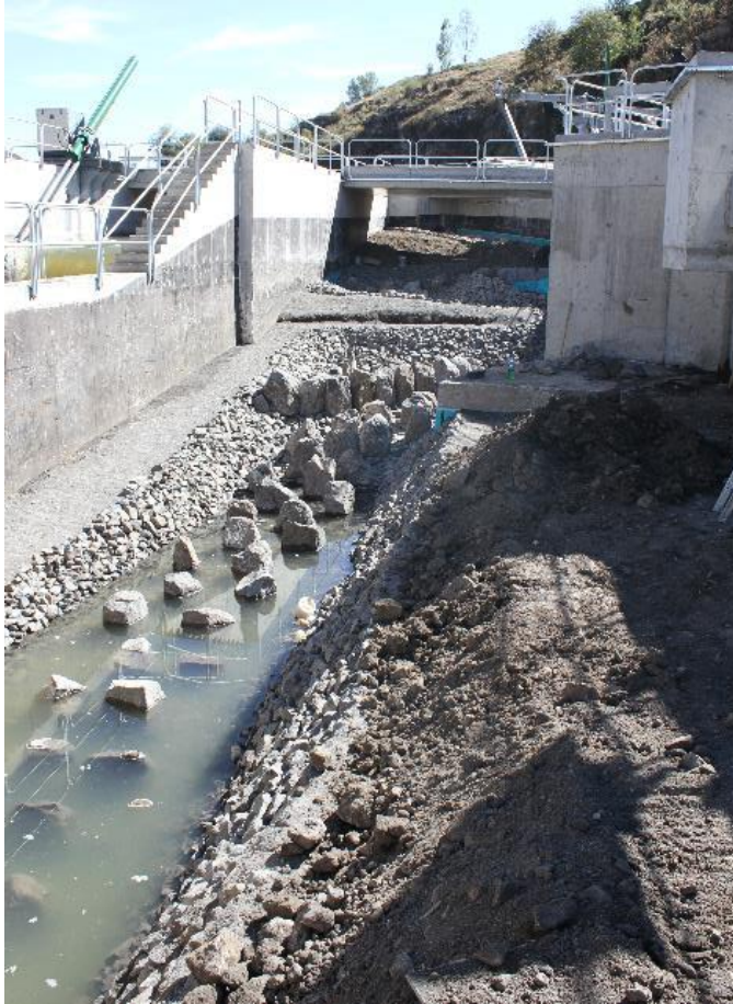
Figure 3.10: Construction of the upstream fish passage at Akhalkalaki 1 ongoing at the time of the visit.
