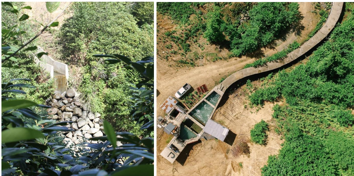
Figure 3.3: Headrace canal covered by concrete slab and forebay (right photo) with forebay spillway located in virtually inaccessible area (left photo), both which reduces health and safety risks.
