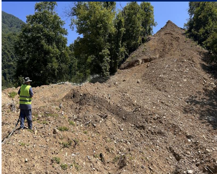
Photo #5: Hydroseeding carried out at HPP area
