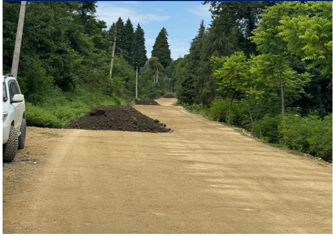
Photo #29: Rehabilitated road in the village of Vaniskedi
