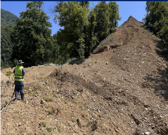
Photo #5: Hydroseeding carried out at HPP area
