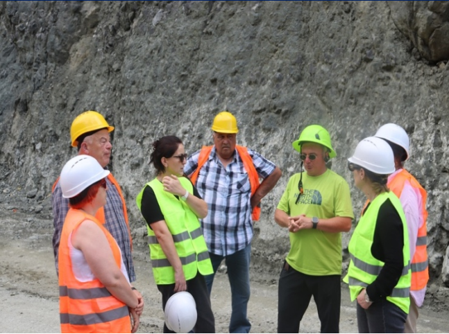
Photo #26: Advisory Council visit at construction site
