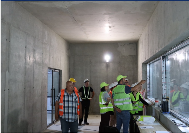
Photo #15: Advisory Council visit at construction site
